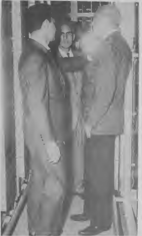
M. E. TROMP, a one-time Lago employee in Electrical, who was one of the supervisors on the new telephone exchange project in San Nicolas, explains intricate equipment to President Murray, center, and PR/IR Manager B. E. Nixon.
